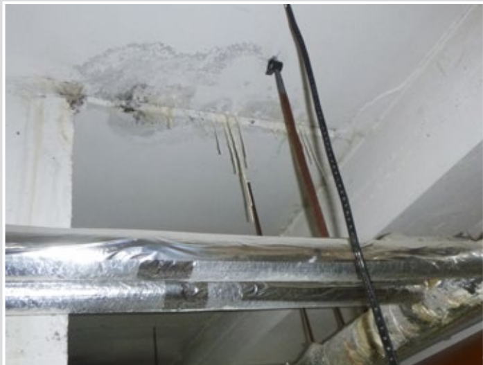
‘Communicating tubes’ without the sealing of the capillaries and water proofing tapes resulting in failures from penetrating moisture to the pool surroundings and/or the lower rooms.
