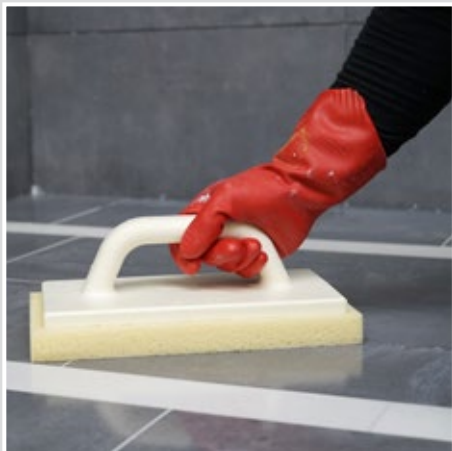
Wash the joints smooth and clean with a hydro sponge board.
