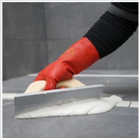
Use the professional board holder to spread the material deep into the joints.
