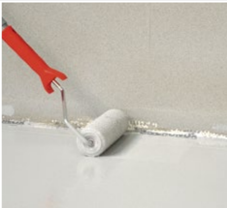
Within 12 - 24 hrs apply the coloured coat of SCHÖNOX EA PUR using a suitable roller.
