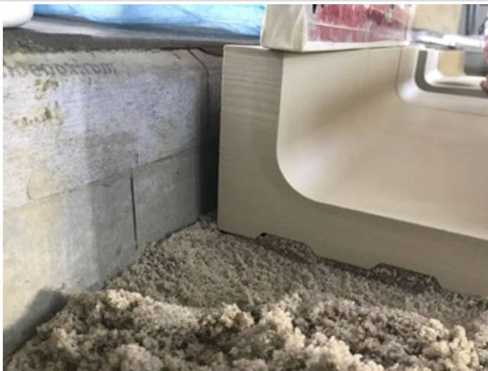
Detail picture of an embedded form part into the aggregated mortar
