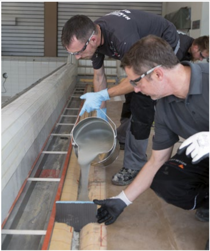
Installing the capillary breaking joint mortar section by section using prepared templates.
