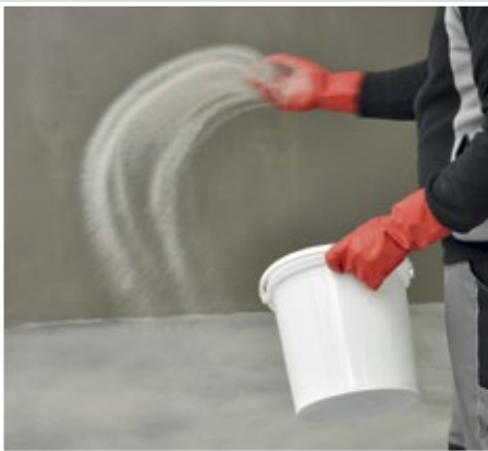
After drying, sand broadcast in excess.
