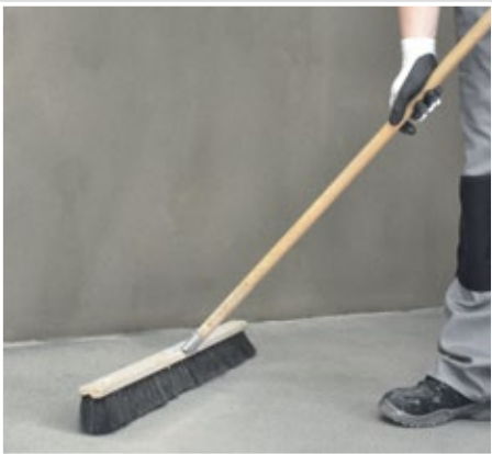
When the epoxy has dried accordingly, broom sweep and vacuum the surface removing any loose sand.
