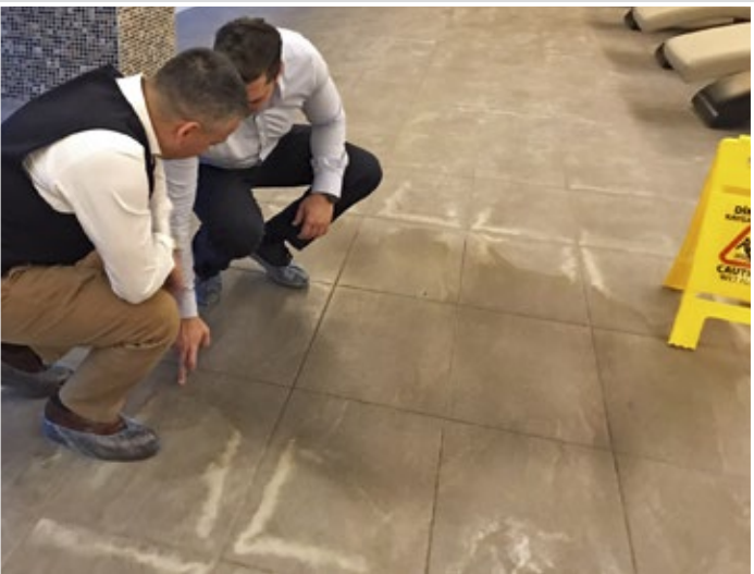
The consequence of insufficient capillary sealing.
