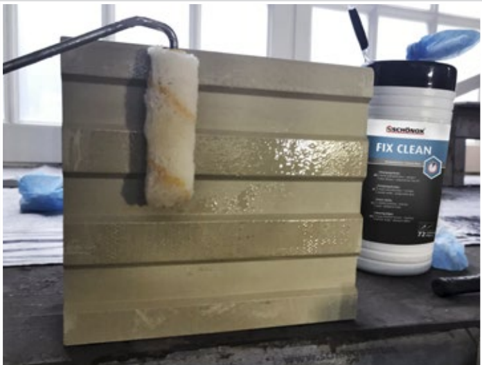
To maximise a suitable bond, the backing of the single components/form parts is primed with neat SCHÖNOX CON BODEN prior to embed into the aggregated mortar.
