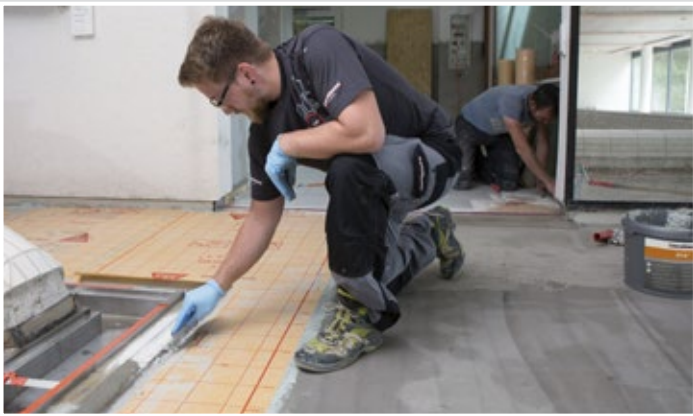
Pressing on SCHÖNOX AB 10/30 around suitable edges.
