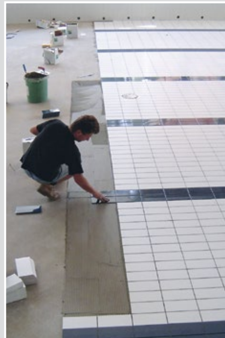
Installing following the floating buttering method resulting in a 'void-free' installation. Picture left: Approving a suitable wetting.
