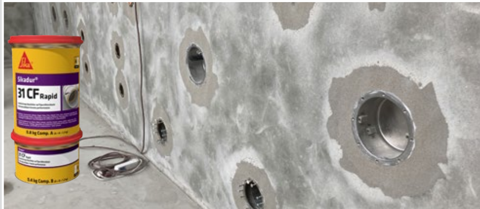
Sample repairs when insufficient flange contact area
