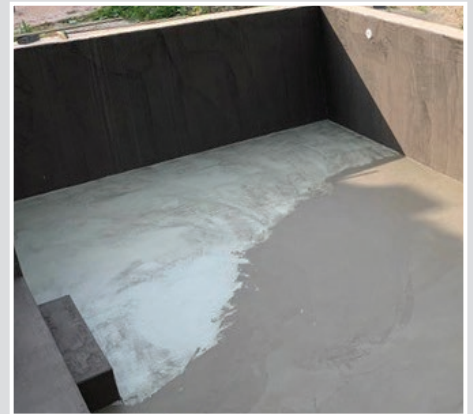
Installation of a cement-based waterproofing system
