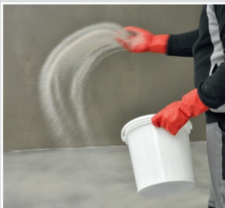
After drying, sand broadcast in excess.
