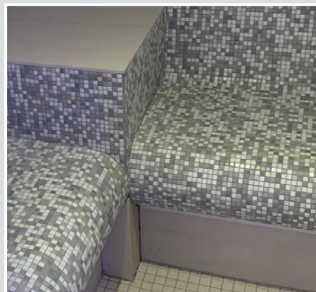
Installing following the floating buttering method resulting in a 'void-free' installation. Picture left: Approving a suitable wetting.
