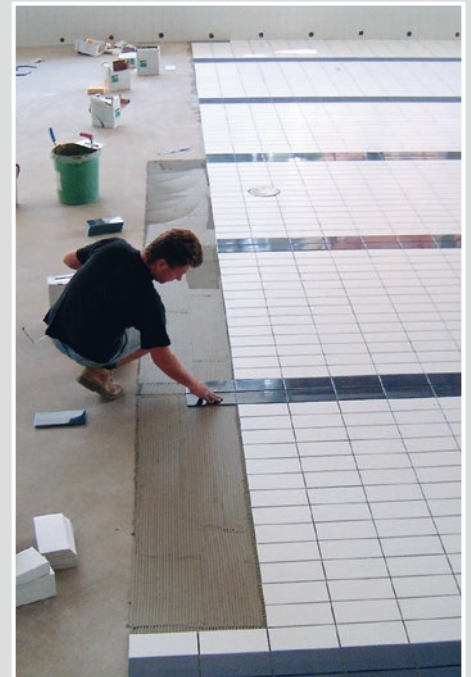
Installing following the floating buttering method resulting in a 'void-free' installation. Picture left: Approving a suitable wetting.
