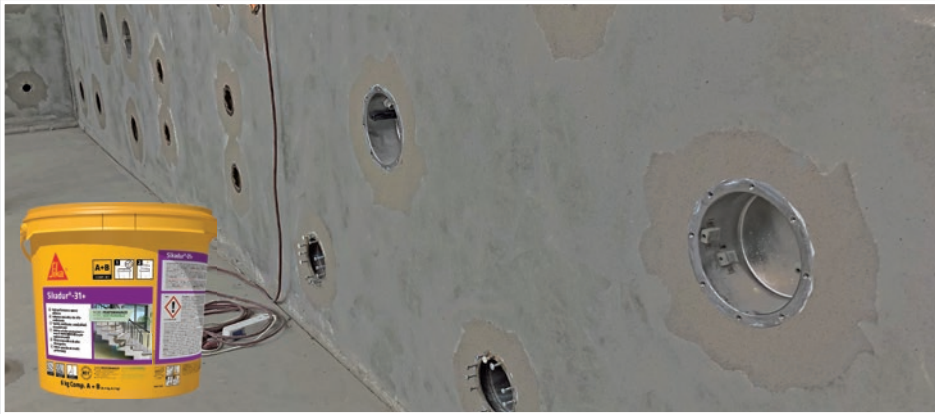
Sample repairs when insufficient flange contact area
