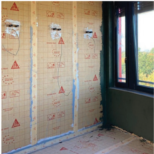
SCHÖNOX AB fullfils the requirements of the W3-I acc. to DIN 18534. The fast curing ensures a prompt utilisation of the sealed area.
