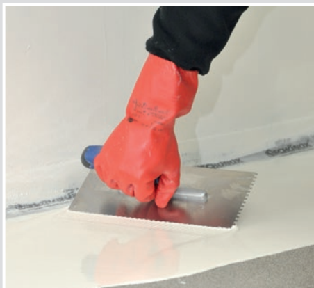
Apply the polyurethane based membrane SCHÖNOX EA PUR / EA PUR S using a 6 mm trowel.
