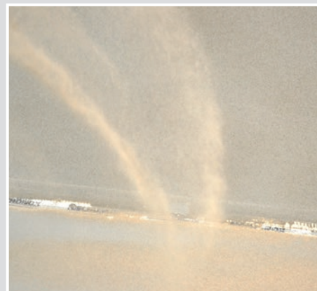
Sand broadcast & cleaning steps again following the product data sheet.
