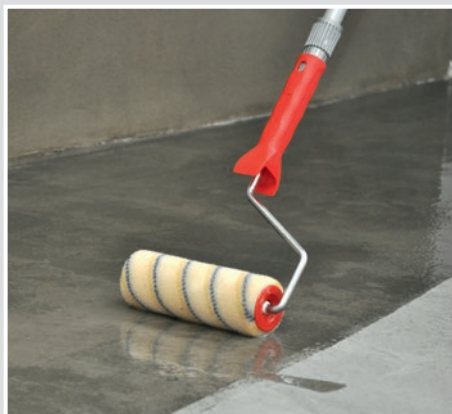
Apply the epoxy based system component primer SCHÖNOX GEA using a suitable, short piled roller following the product data sheet.
