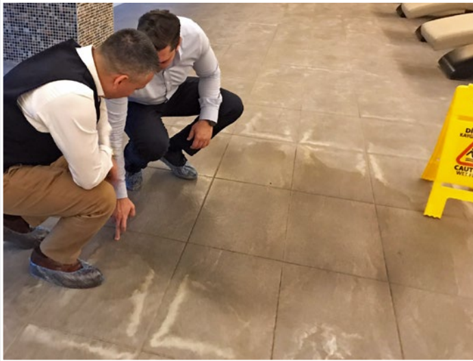
The consequence of insufficient capillary sealing.
